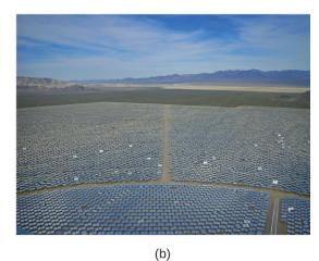
**Figure 5.10** (a) The Ivanpah solar thermal plant uses 170,000 mirrors to concentrate sunlight on water-filled towers. (b) It covers 4000 acres of public land near the Mojave Desert and the California-Nevada border. (credit a: modification of work by Craig Dietrich; credit b: modification of work by "USFWS Pacific Southwest Region"/Flickr)
